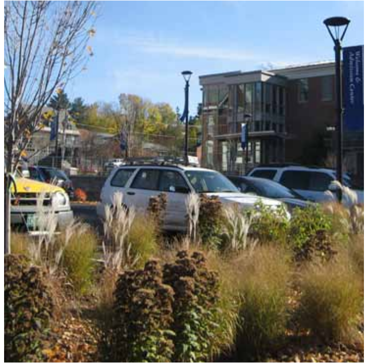
Above, bioswale adjacent to parking area at Champlain College collects and retains stormwater from the adjacent parking lot and allows it to infiltrate through the soil.
